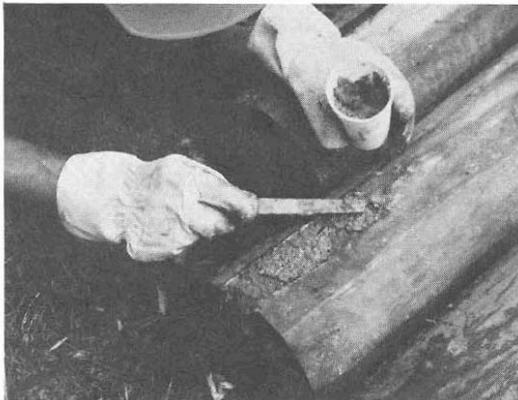
*Epoxy can be used to spot-repair damaged areas on a log.*
