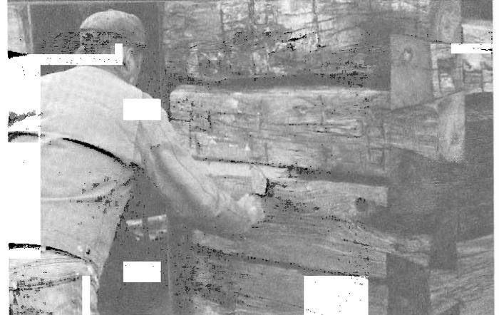
*Mortar applied with a trowel seals the seams between logs.*
