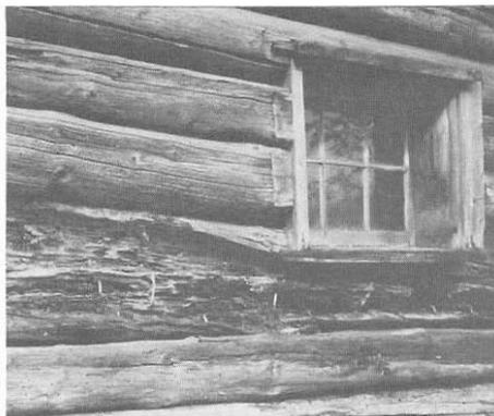
*This log, damaged by both water and insect infestation, needs to be replaced.*
