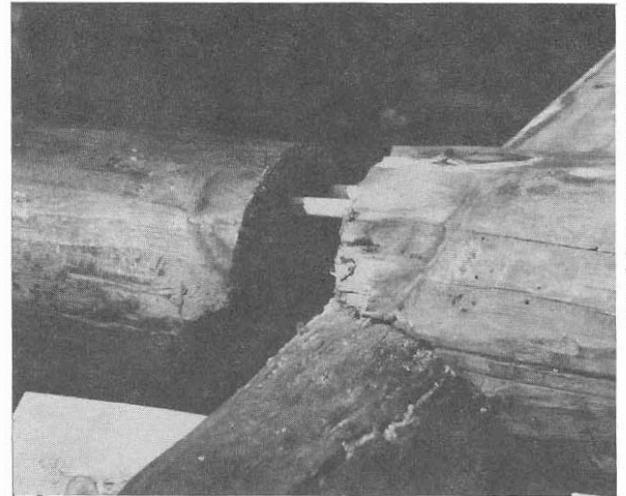
*Fiberglass rods secure a replacement crown.*
