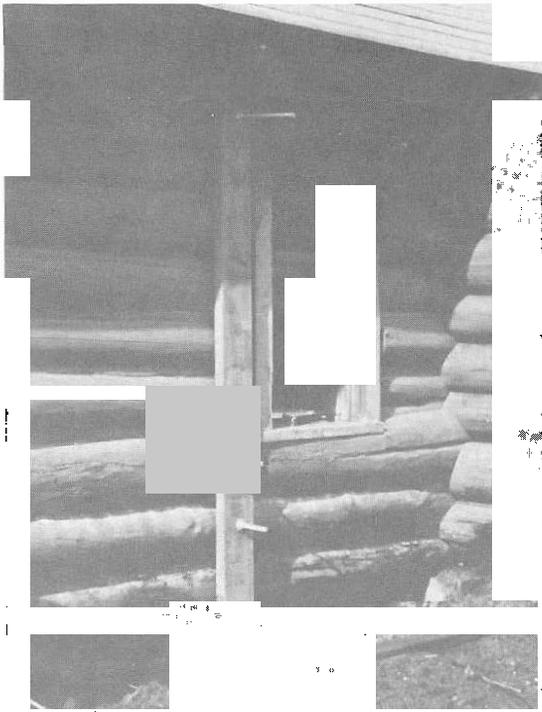
*Vertical supports called cribs stabilize the wall before it is lifted to make way for the replacement log.*
