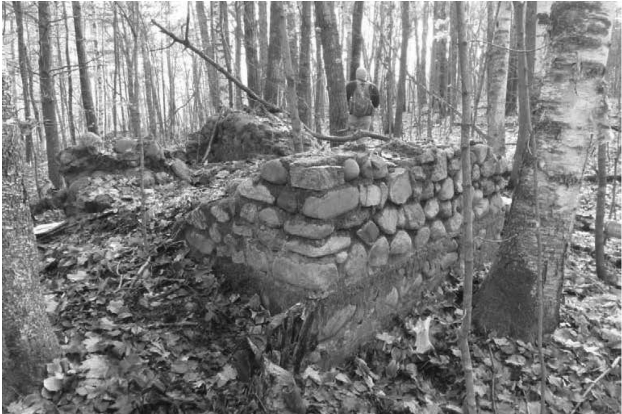
Remainder of stone fireplace chimney at CCC Camp S-142 in Becker County. The camp was in operation from 1934 to 1935. The chimney was documented as part of the Statewide Survey project "Documenting Minnesota's CCC Camps."
